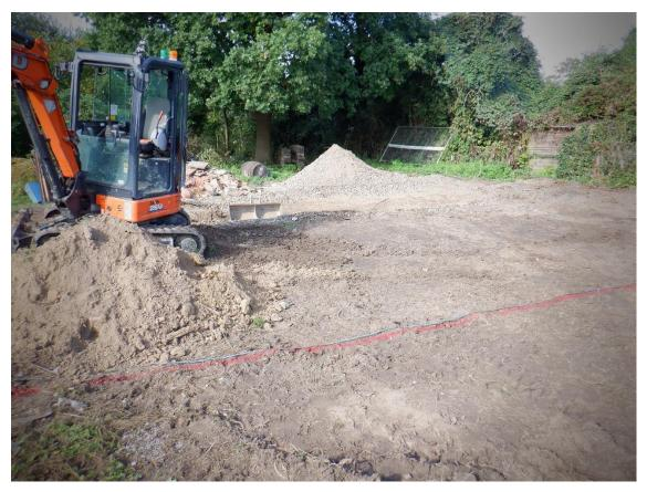
Plate 1. Setting out and starting ground reduction (looking SW)
